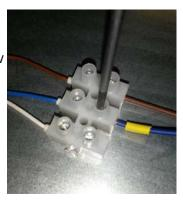
Disconnect the heat demand cable from the control panel (taking note of its terminal number) and join to the new **WHITE** wire using the terminal block provided.
