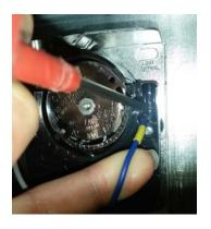
Remove the old fan/limit stat by removing the fixing screws and fit the replacement.
